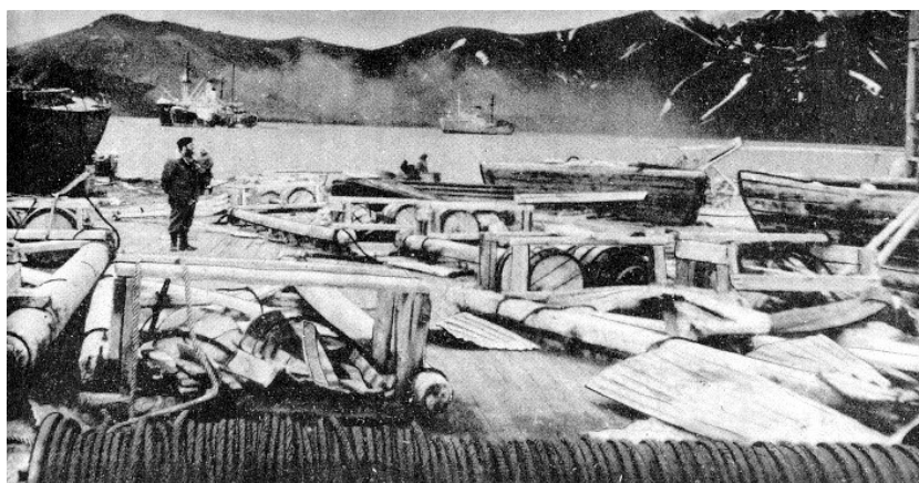
Figure 10. Construction work at what is today the Captain Arturo Prat Antarctic Naval Station. Source: Terra Australis , Eugenio Orrego Vicuña (1948).
