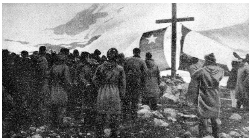
Figure 7. A record of the installation of the first Chilean cross in the Chilean Antarctic Territory. Source: Terra Australis, Eugenio Orrego Vicuña (1948).
