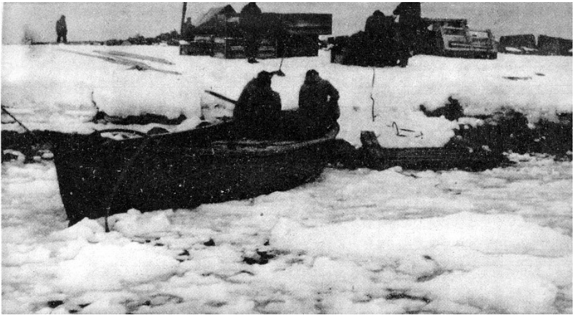
Figure 4. A record of the First Chilean Antarctic Expedition during the construction of what is today the Captain Arturo Prat Antarctic Naval Station. Source: Terra Australis, Eugenio Orrego Vicuña (1948).
